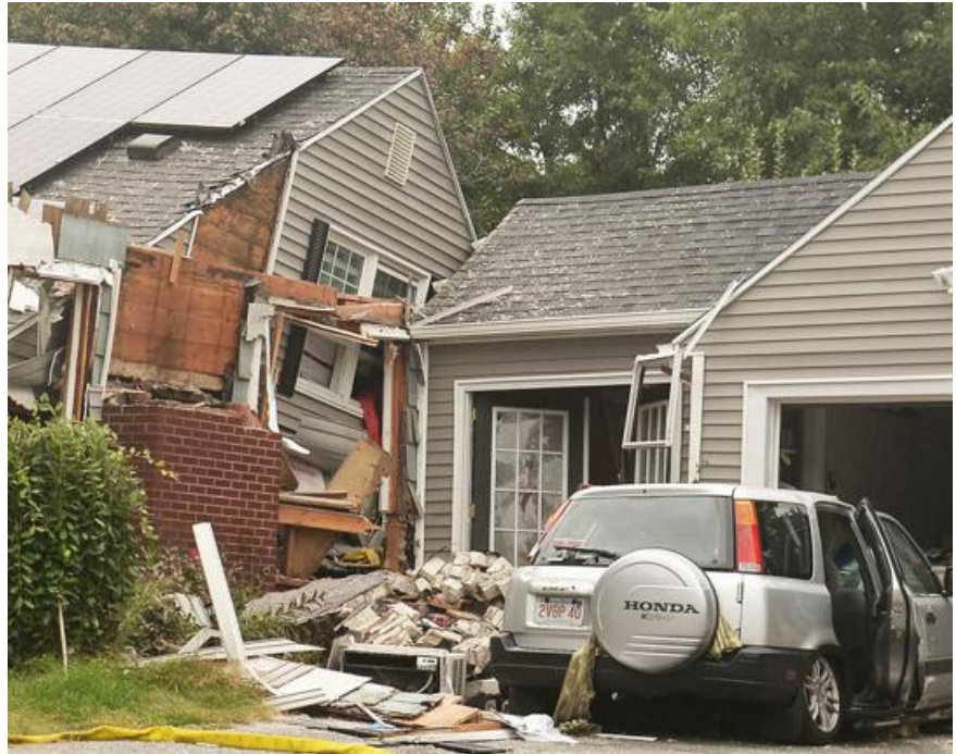
A gas explosion destroyed this house on 39 Chickering Rd. in Lawrence killing Leonel Rondon, 18 when the chimney, seen here, fell on the car he was in.
